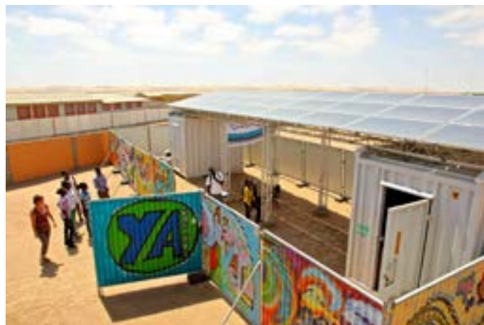
Figure 6.4 YA Namibia - Mobile solar energy station up and ready for use
