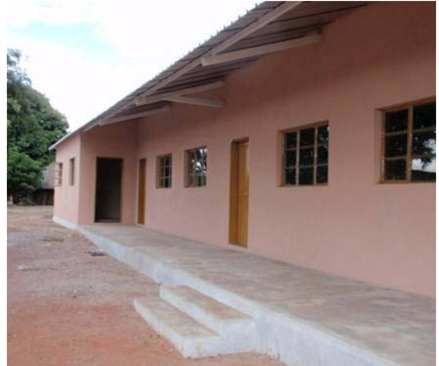
School at Nhatarara after Mozfoods CSR Project
