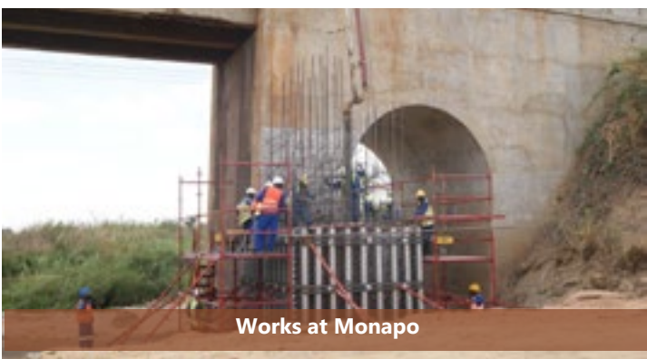
Wingwall shuttering works
