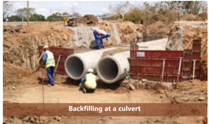
Casting concrete at a culvert
