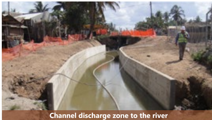
Wall concreted
