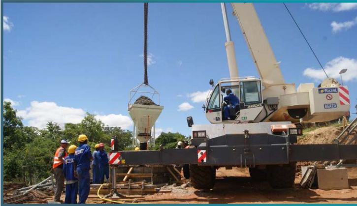
Concrete works at Nagive Bridge
