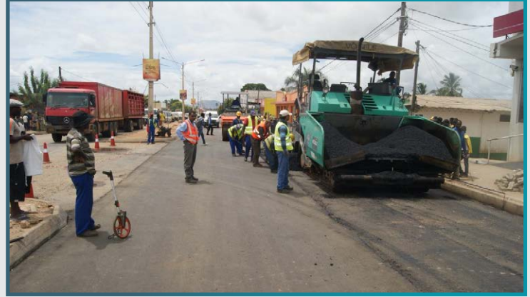
Asphalt works at urban section
