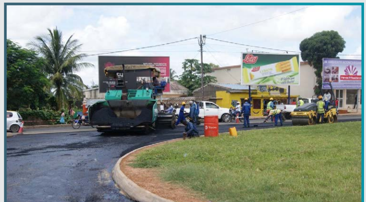
Asphalt works at Airport roundabout
