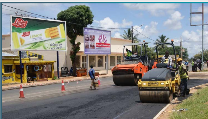
Asphalt works at Airport roundabout
