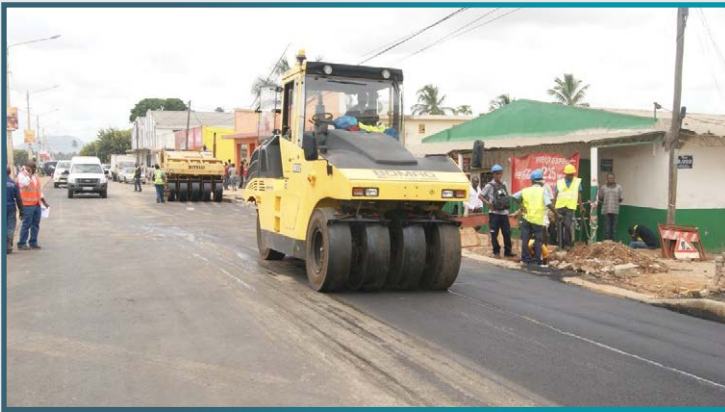
Pneumatic roller Compacting the asphalt wearing course
