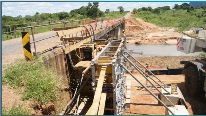
Concrete works at Nagive Bridge
