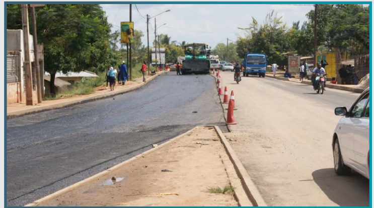
Urban Section asphalt works
