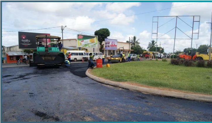
Asphalt works at Airport roundabout
