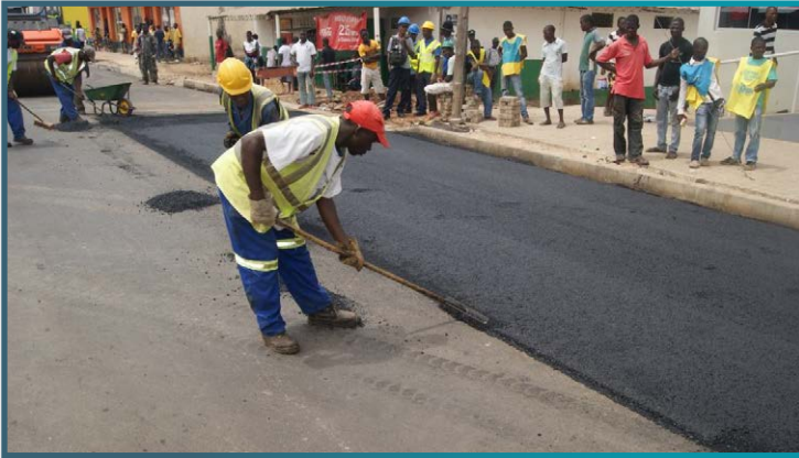
Asphalt works at urban section
