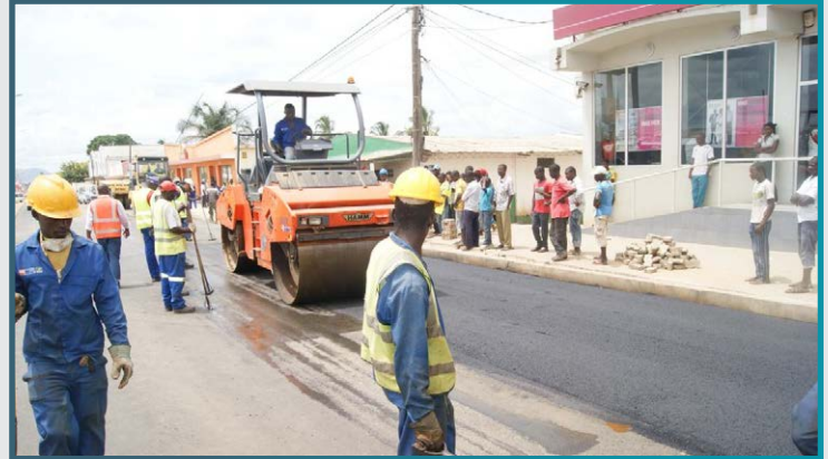
Compacting of asphalt wearing course
