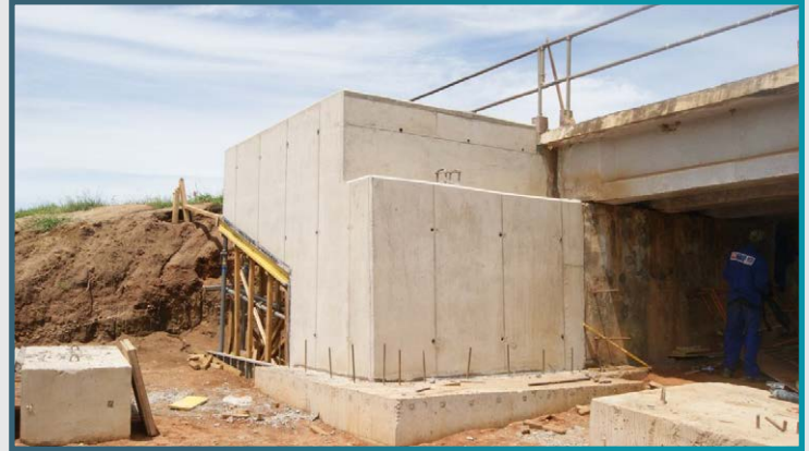
Concrete already casted on Abutment
