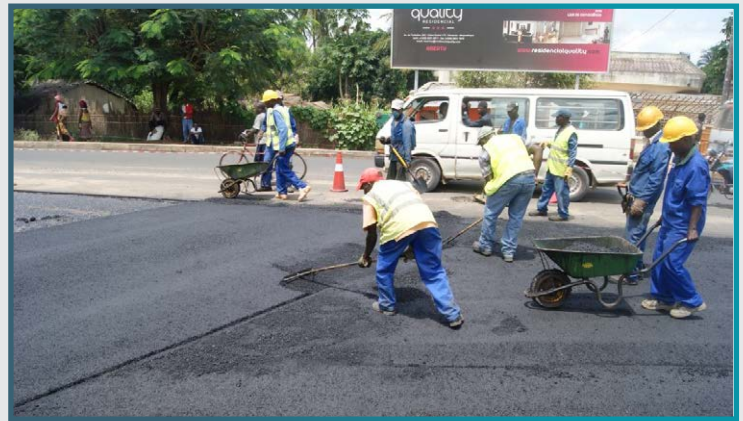
Asphalt works at Airport roundabout
