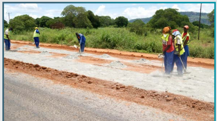
Asphalt works at Airport roundabout during night shift
