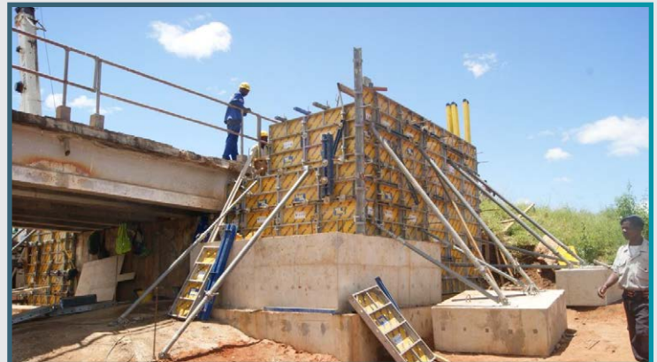
Concrete works at Nagive Bridge
