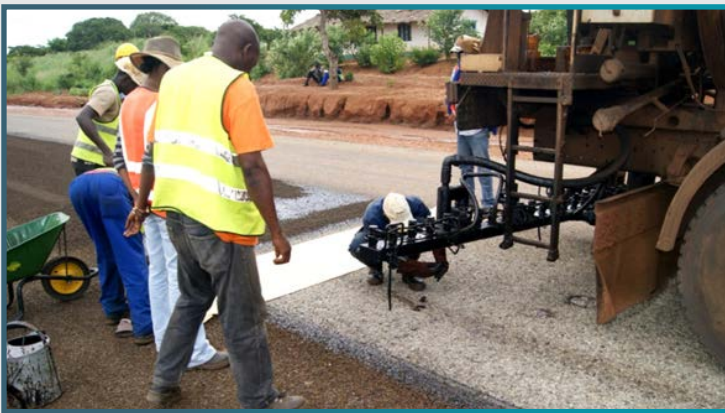
Asphalt works at Airport roundabout during night shift
