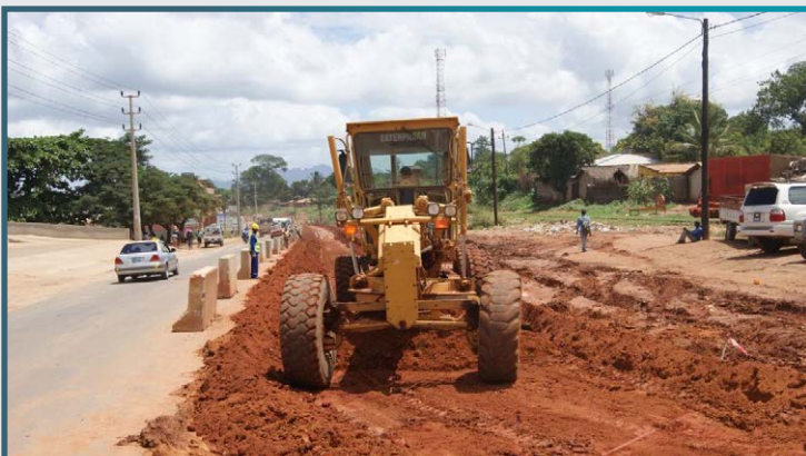
Widening of urban section
