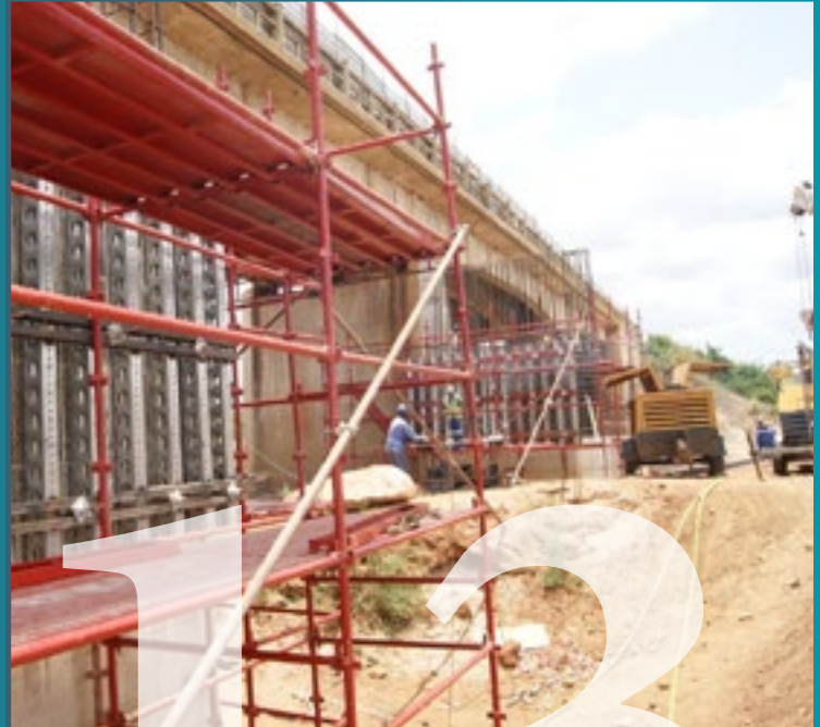
ROADS REHABILITATION PROJECT
