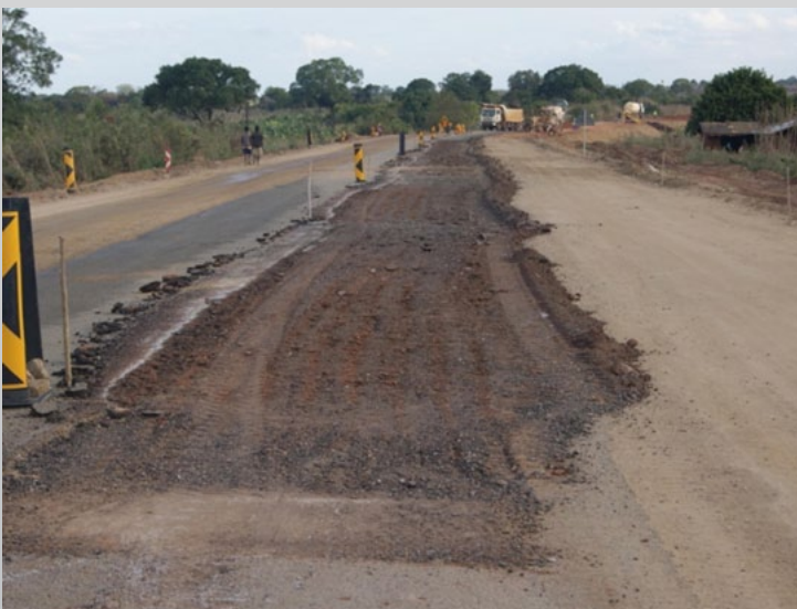
Preparation for subbase stabilization (31th July of 2012)
