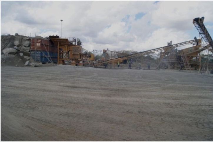
Crusher plant at Namialo Quarry (10th July of 2012)
