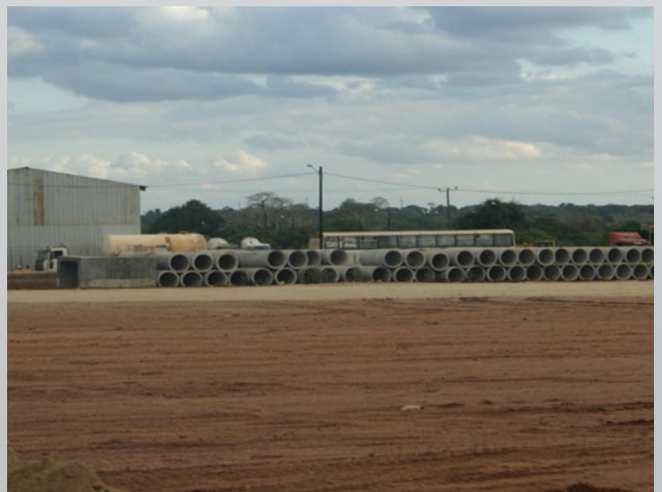
Pipe culverts (31th July of 2012)
