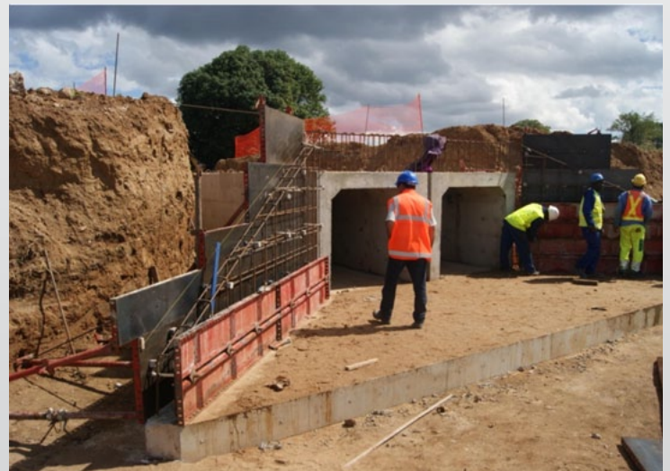
Shuttering of culverts wing walls (10th July of 2012)
