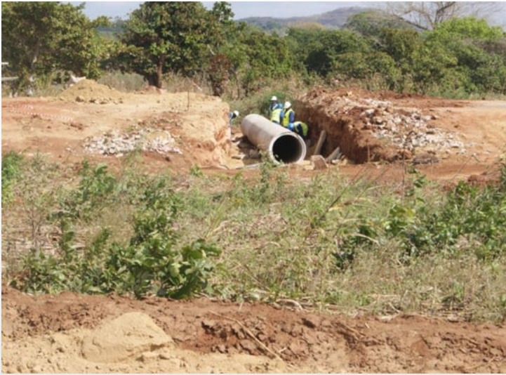
Assembling of a pipe culverts (20th July of 2012)
