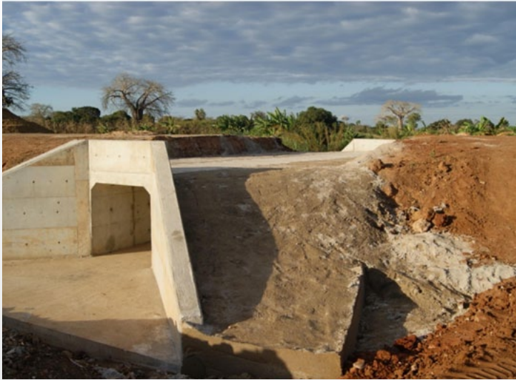
Backfilling of culverts using soil-cement mixture (10th July of 2012)
