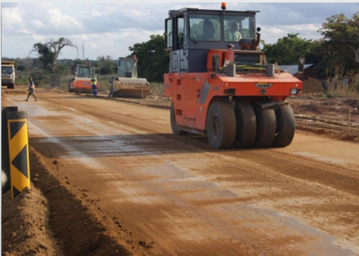
Compacting cement stabilized subbase (31th July of 2012)
