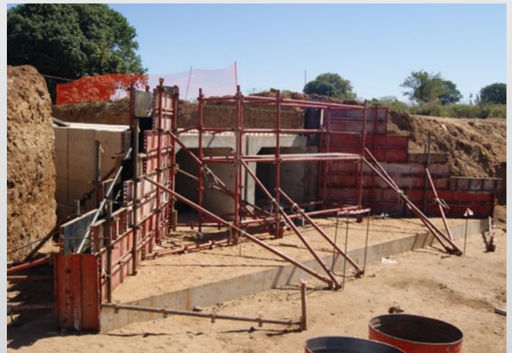
Culvert portals with joints already sealed (13th July of 2012)
