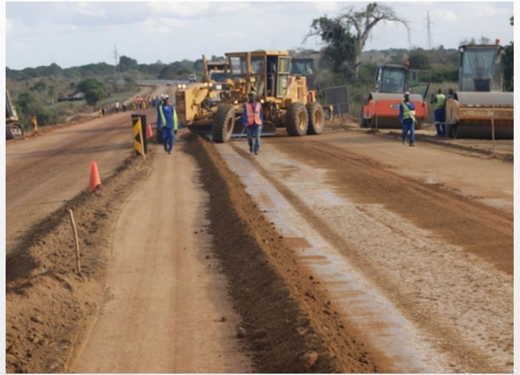
Cement stabilization of subbase (31th July of 2012)
