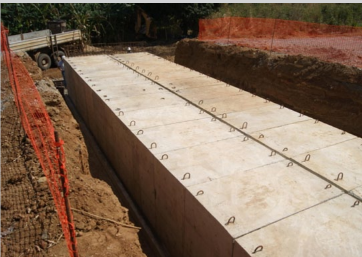
Culvert portals already assembled (10th July of 2012)
