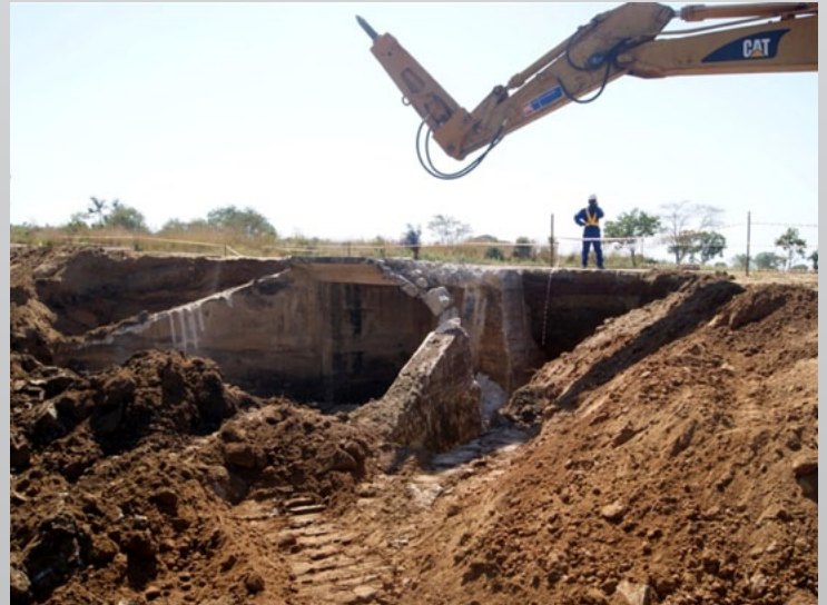
Demolishing of a culvert (16th July of 2012)
