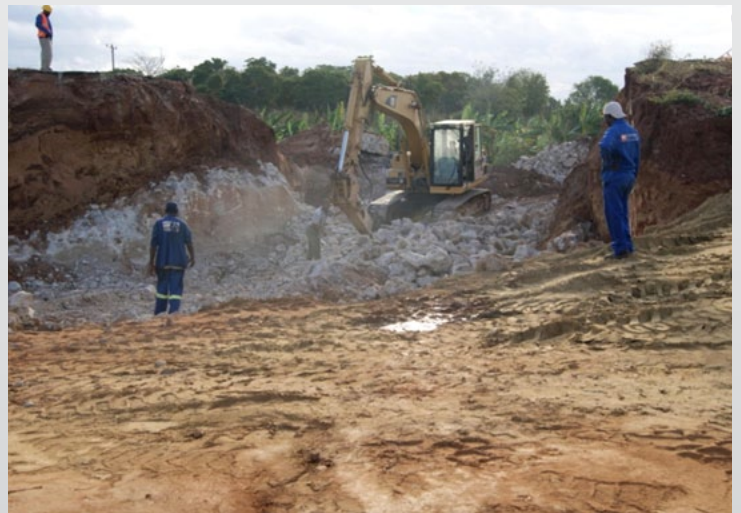
Demolition of a culvert (31th July of 2012)
