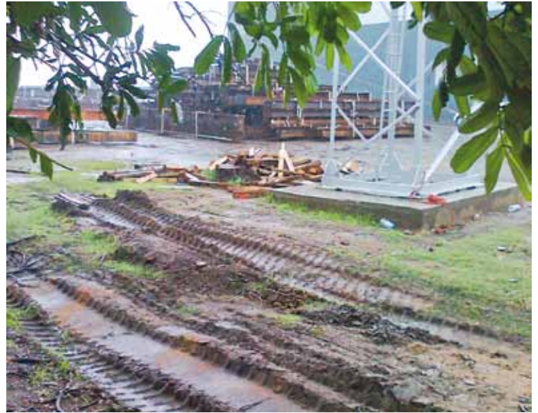
Rain, rain and more rain nearly bogged down the project.
