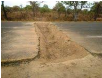
One of the trenches dug into the EN1 near Muxungue
