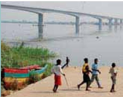
Image 9: Zambezi River Bridge
